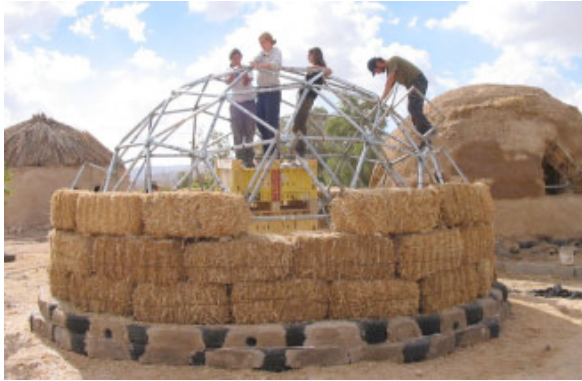
Students constructing a straw bale and earth geodesic dome
